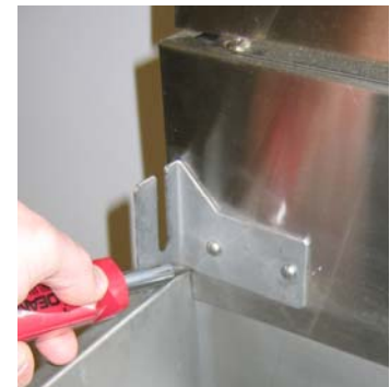
Removing flue cap.
