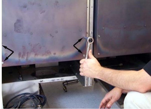
Removing bolts (arrows) securing flue to cookpot.
