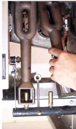
Removing burners from rethermalizer.
