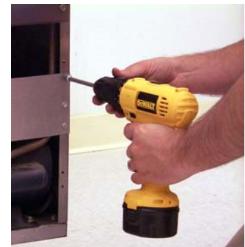
Removing gas manifold shield.
