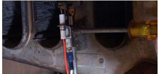
Removing electronic/standing pilot assembly.
