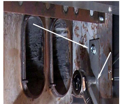
Removing bolts (arrows) from burner manifold support brackets (both sides). Leave the burner manifold in place after removing bolts.
